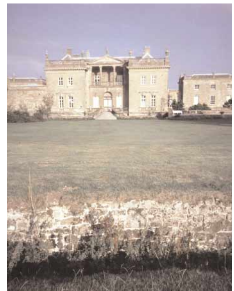
BELOW: Front lawn of manor house at Stourhead, showing the ha ha wall.
